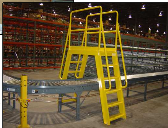
Crossover and emergency stops at NE corner of system.
