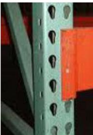
**THE BEAM ENDPLATE:** While there are literally dozens of variations, the most common beam endplate style today is teardrop, with slotted and bolted also retaining popularity. The one common element is safety locking the beam to the upright, preventing it from being knocked out. Because beam locks vary by manufacturer, it's good practice to ensure your beams match your uprights.
